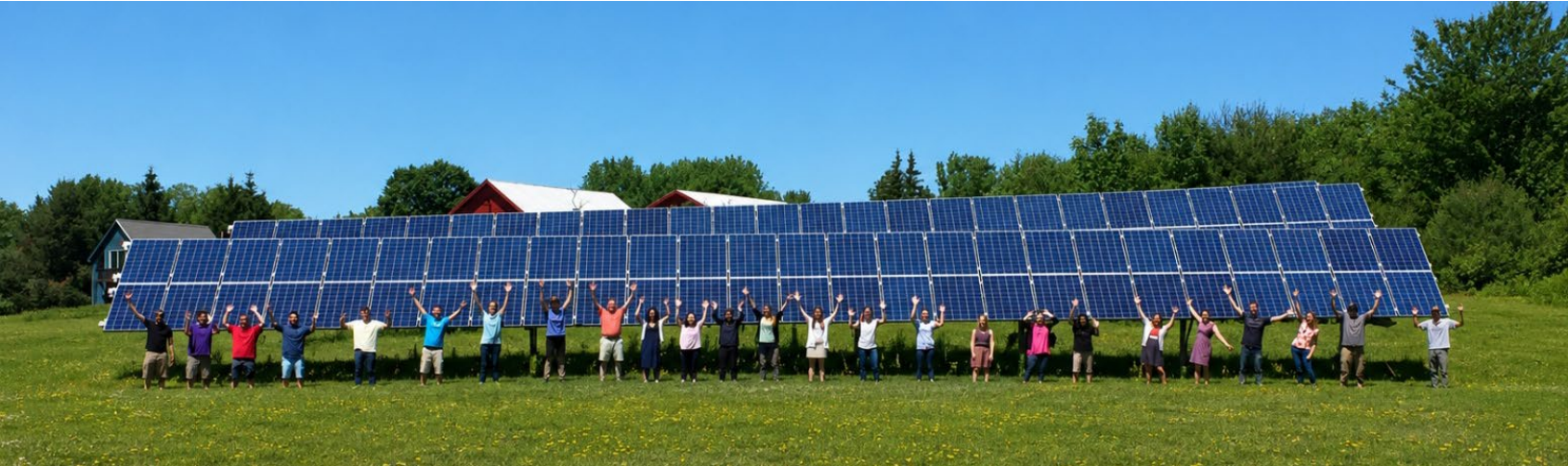
Planson HQ: Employees stand in front of on-campus solar arrays
